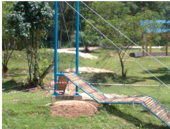
Fig. 6 A simple pedestrian suspension bridge
