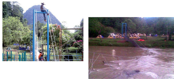
b) Collapse of Kuala Dipang suspension bridge
