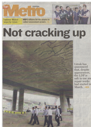
c) Crack repairs in flyovers at Puchong Jaya
