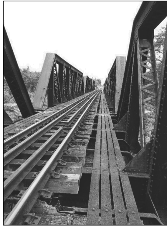
Figure 10 The connection and jointing system at the inner truss is more complicated than outer truss
